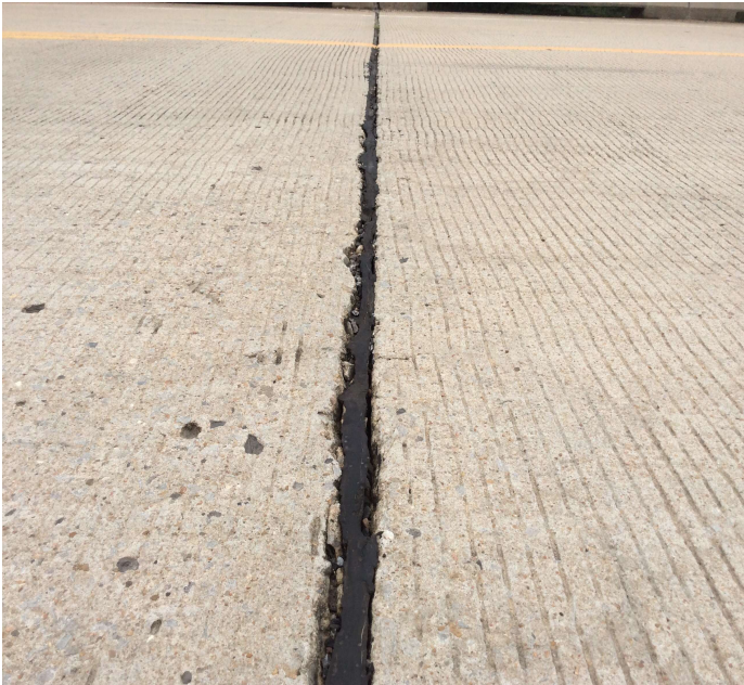
PHOTO 1 Description The deck joints seals are deteriorated and leak water.
