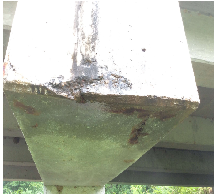
PHOTO 2 Description There are two delaminated areas in the Rt end of Bent 4 cap.
