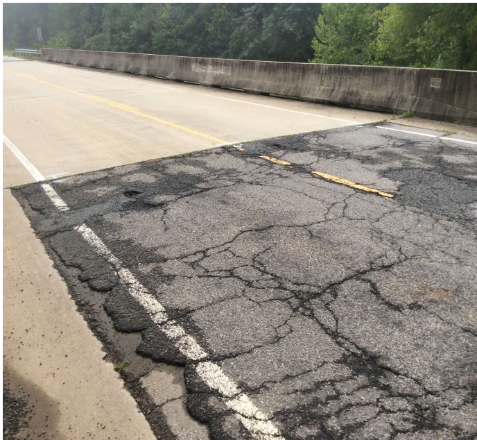
PHOTO 1 Description Minor asphalt settlement at the approaches.
