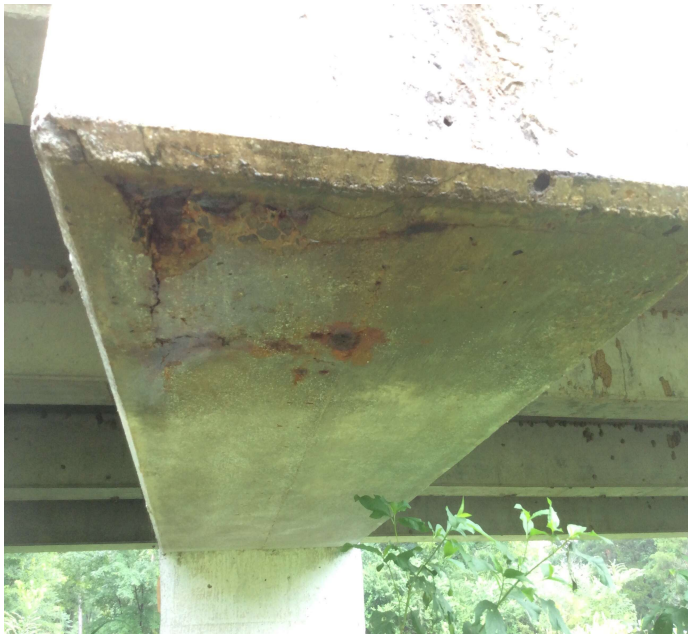
PHOTO 1 Description Spalling with exposed reinforcing steel on the under surface of the cap at Bents 2.
