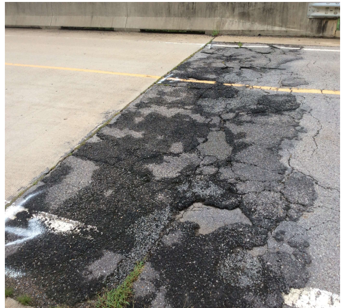
PHOTO 2 Description Minor asphalt settlement at the approaches.
