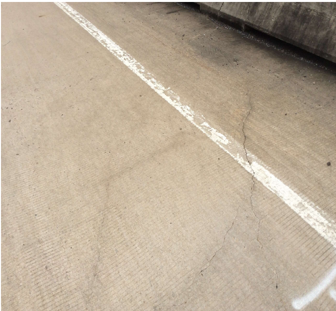
PHOTO 1 Description Sealable cracking on the driving surface of the deck.
